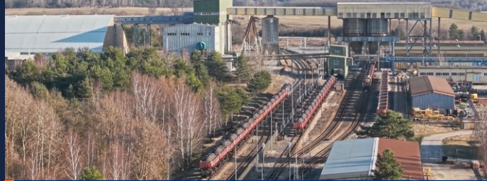
Rail loading yard at the smelter
